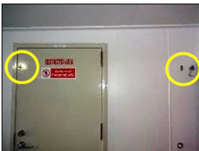
Hold-back hook fitted on self-closing door
