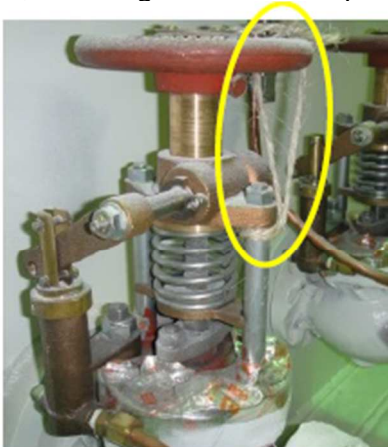
Quick closing valve lashed by rope
